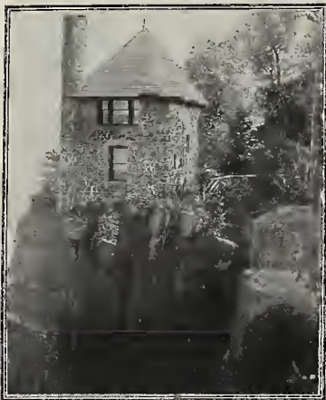
THE NORDHOFF TOWER.
